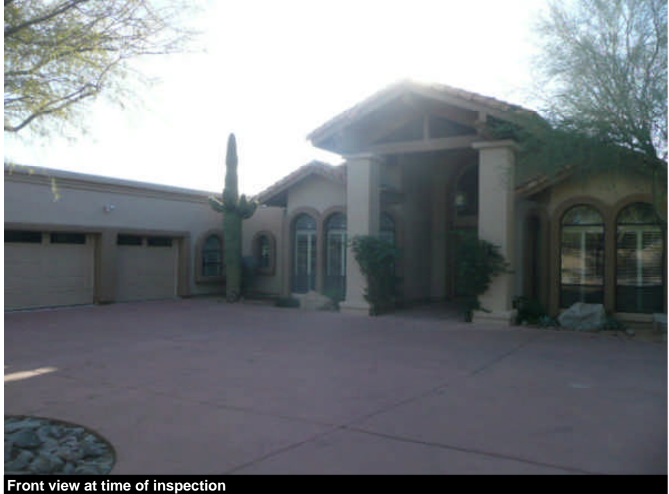
Front view at time of inspection
