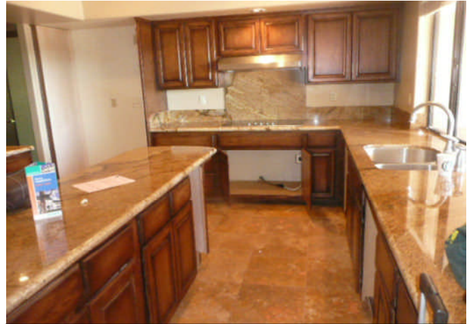
Kitchen view and condition at inspection
