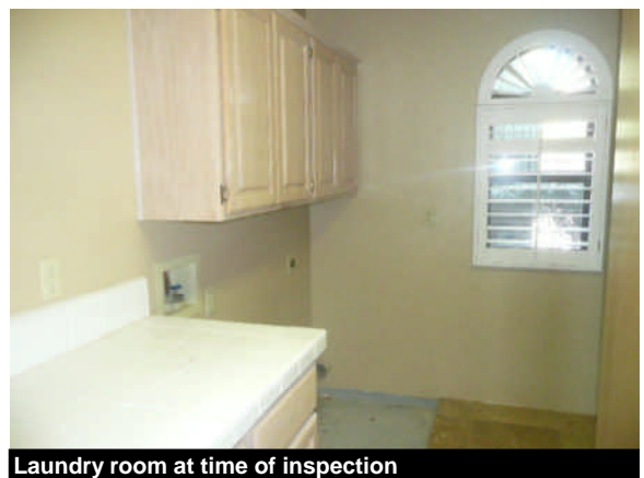
Laundry room at time of inspection
