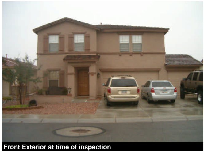
Front Exterior at time of inspection
