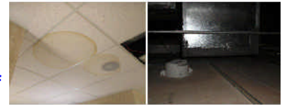
Missing ceiling tile
