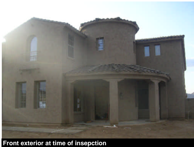
Front exterior at time of inspection
